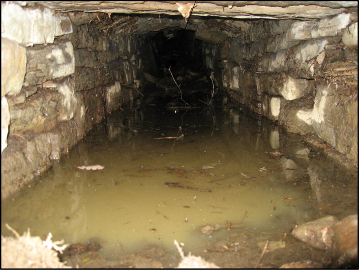
Photograph of the culvert
