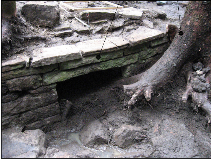
Photograph of the down stream culvert exit during excavations, now backfilled
