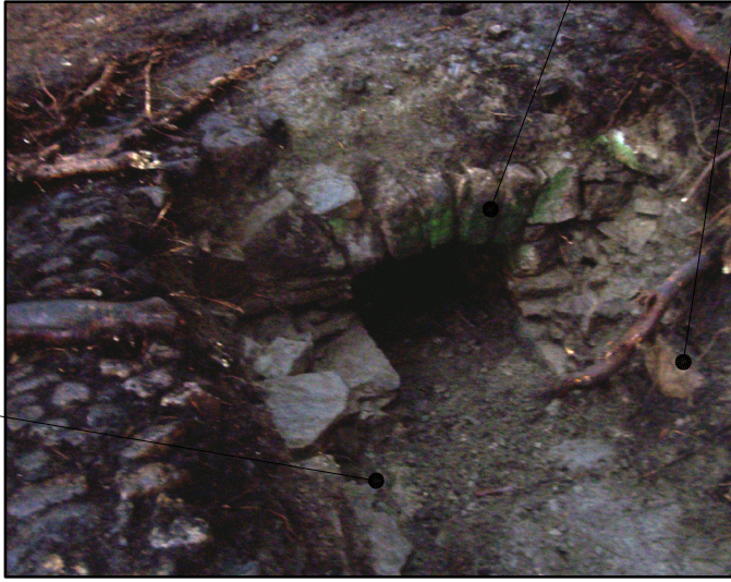
Photograph of the upstream culvert entrance during excavations, now backfilled
