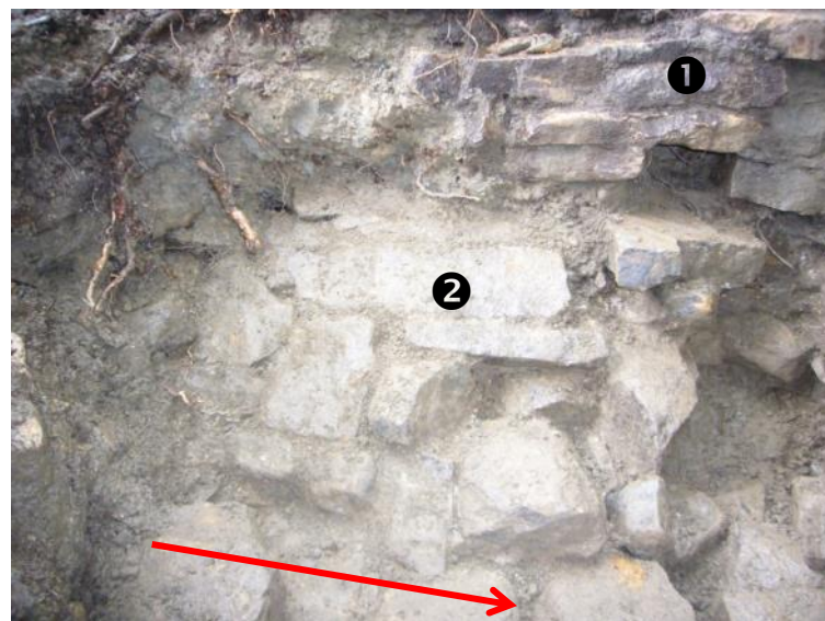
Figure 14. Possible Revetment in Leat Bank
