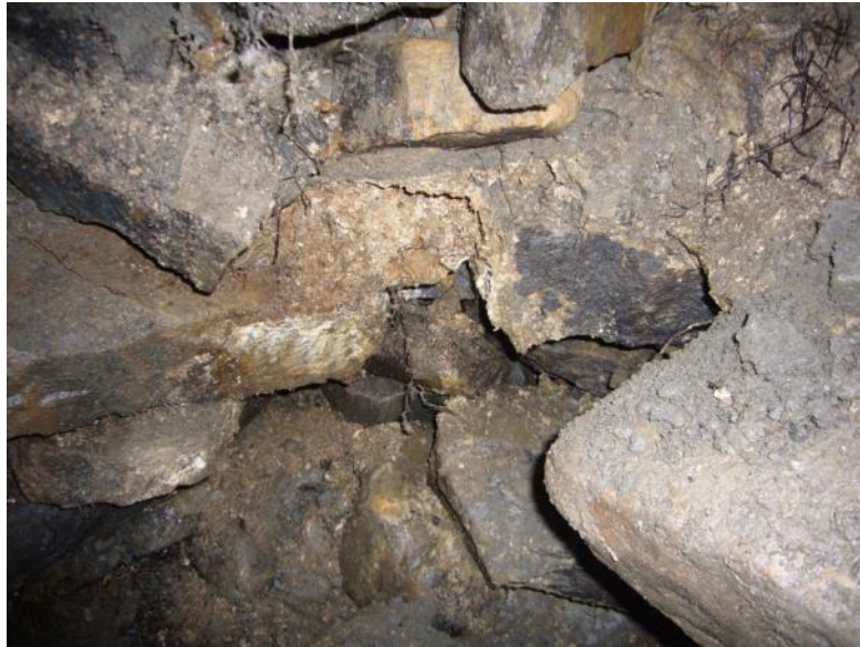
Figure 11. Close-up of In-fill Stones
