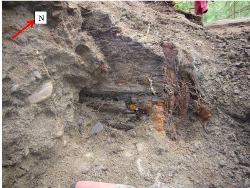
Figure 2. Shuttering and Vertical Post
