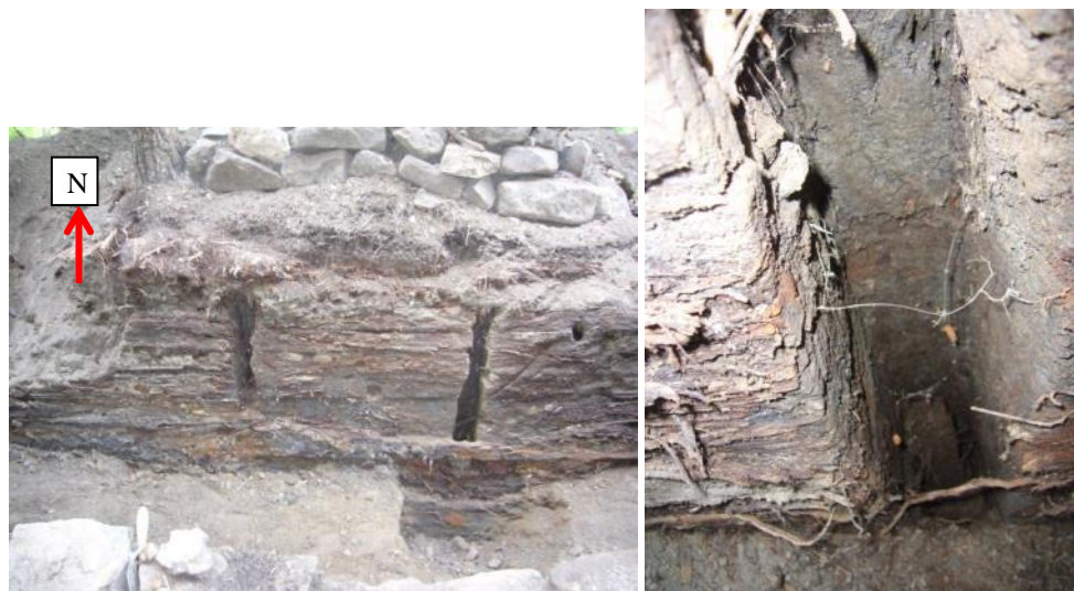
Figure 12. Slots in Shuttering
