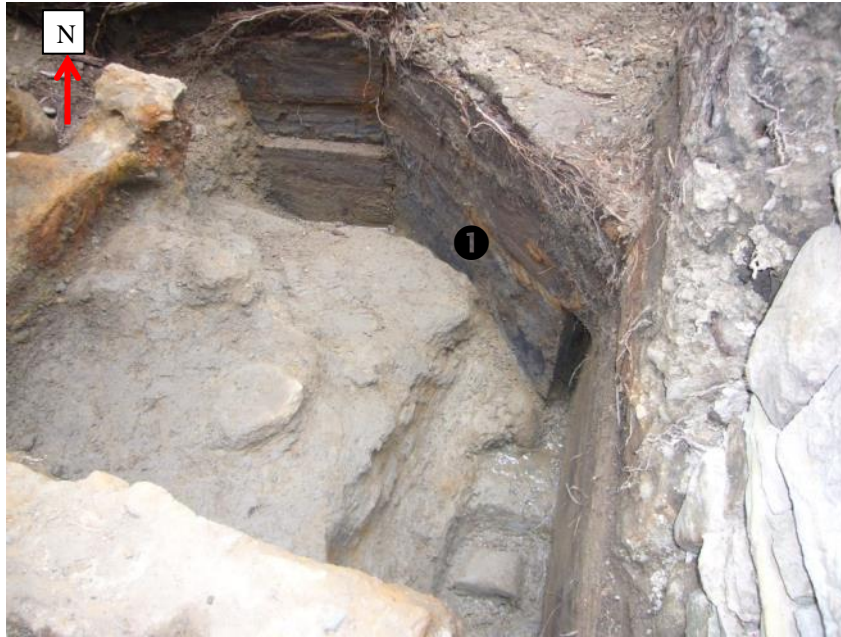
Figure 10. Bottom of Shuttering, Culvert End of Mill Pond
