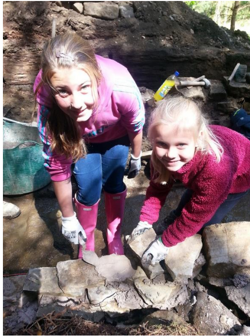
Pupils from Allendale Primary School consolidating the leat with lime mortar
