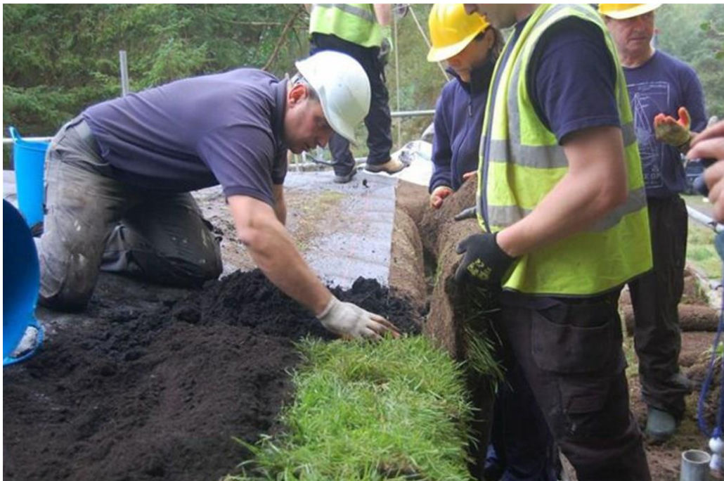
Applying soil and turf onto the membrane on top of the arches
