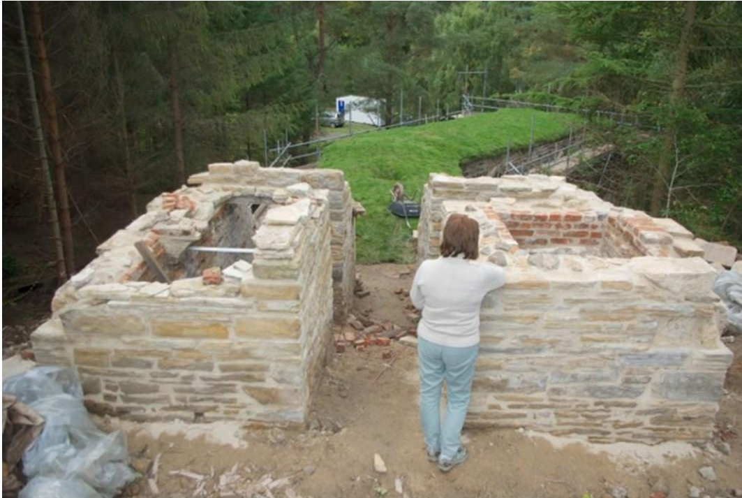
Chimneys repointed, soft capping completed
